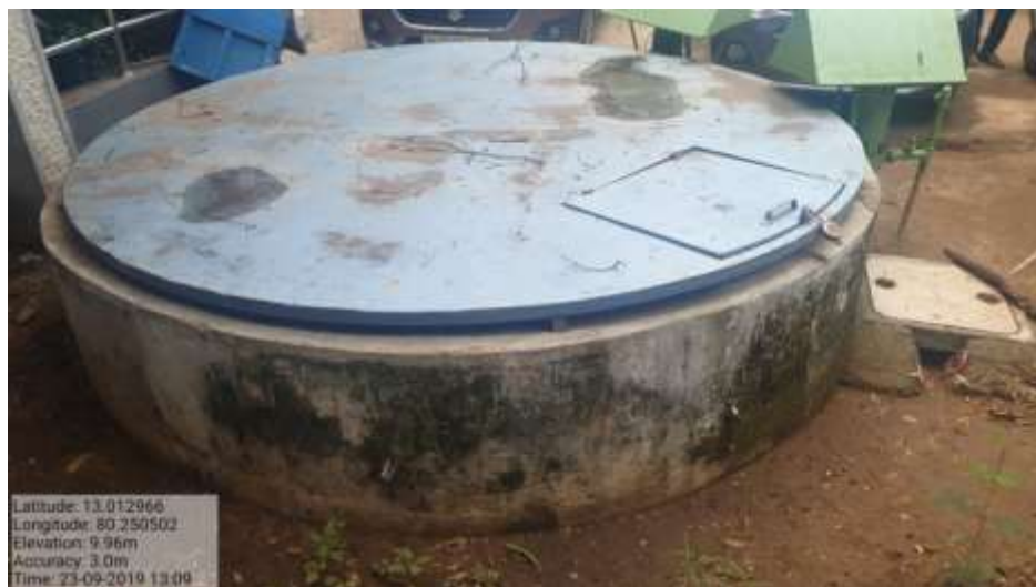
Plate 18: Rain Water Segregation Chamber – D Block
