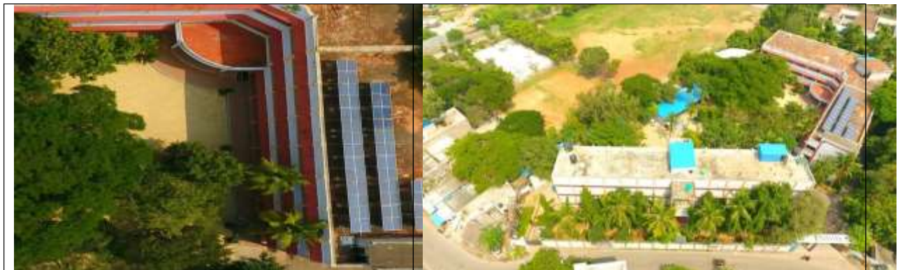
Bird's Eye View – Solar panels
